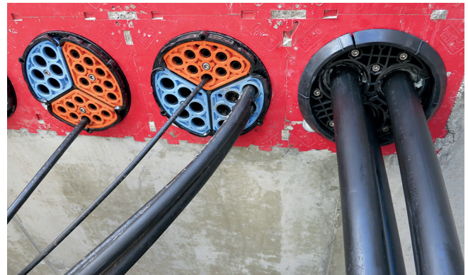
Sealing with Segmento and HSI 150-DG.
